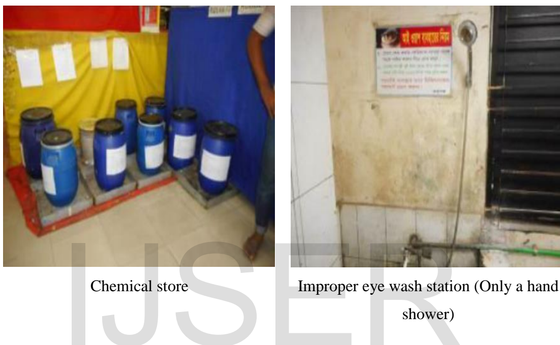
Fig. 4.25 Chemical store and improper eye wash station in the chemical handling area
