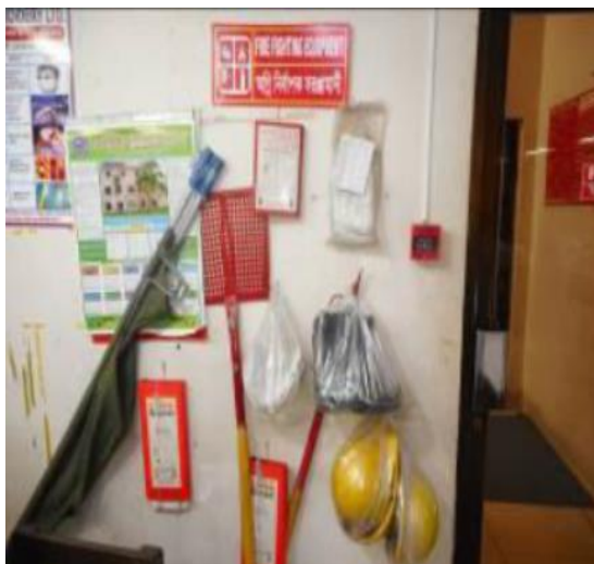
Fire alarm switch
